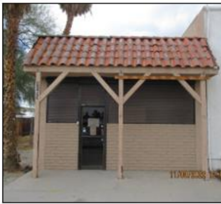
Prior to Building Improvements
